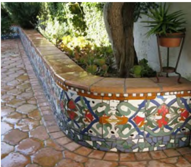
TILE INLAY SEAT-WALLS
