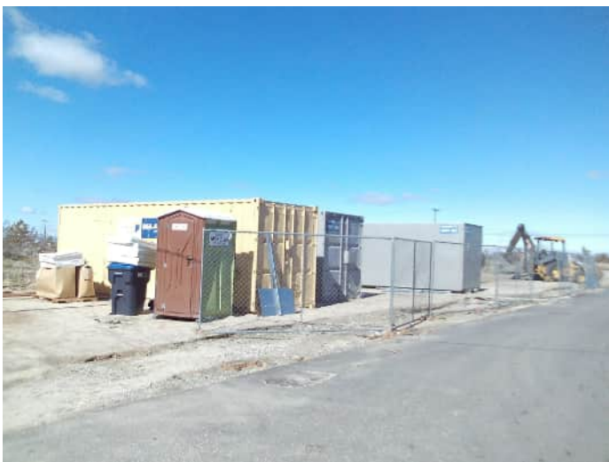
17. View of construction equipment on the east adjoining property
