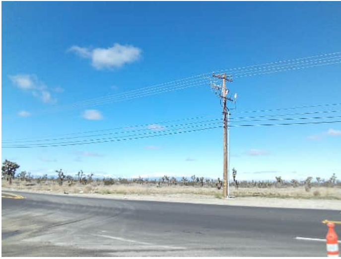
19. View of the north adjoining property from across East Palmdale Boulevard
